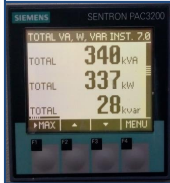
Energy Meters with real time communication to DCS.
